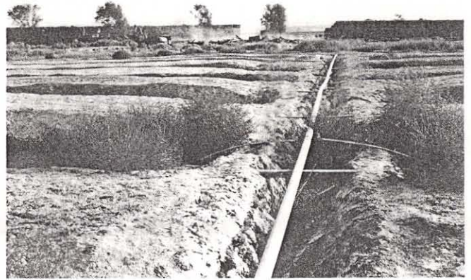
Figure 8. Header pipe used to supply geothermal water to ponds.
