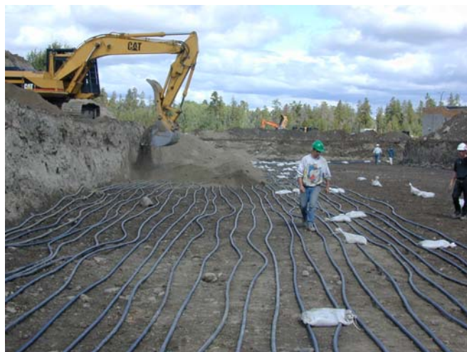
Figure 6. This photo shows the installation of the horizontal earth loop at 100 Mile House, BC. 50,000 feet (15,200 m) of 1 inch (25 mm) pipe was installed to a depth of 8 feet (2.4 m).
