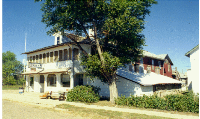
Figure 7. Stroppel Hotel in Midland. The baths are located under the sloping roof structure on the right.
